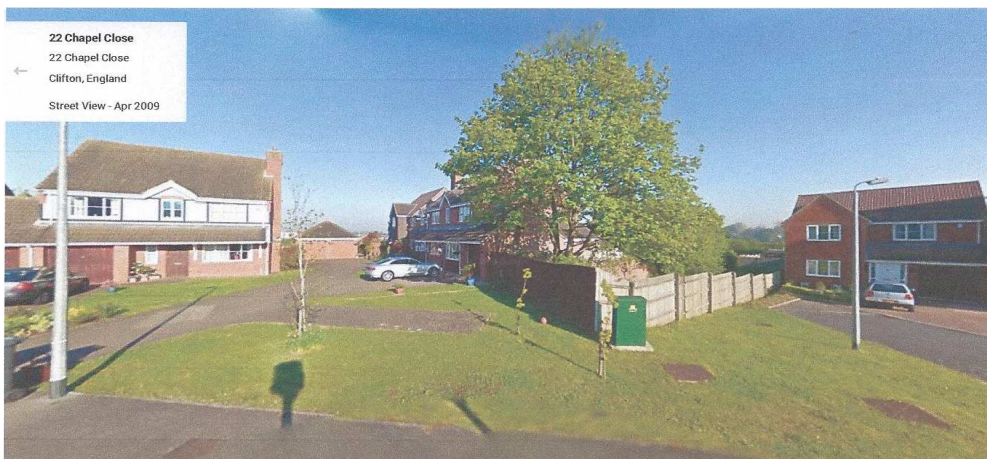
Street scene in Chapel Close prior to the development of 11 new houses by the applicant in 2013/14
